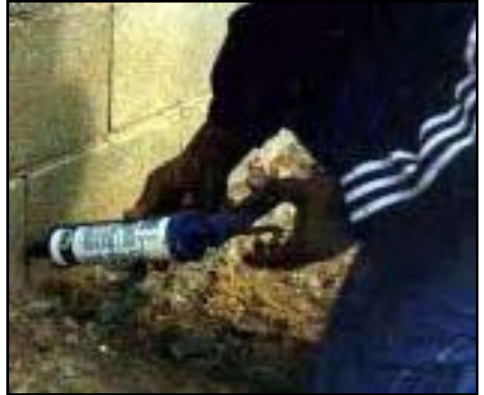
Seal holes with caulk
