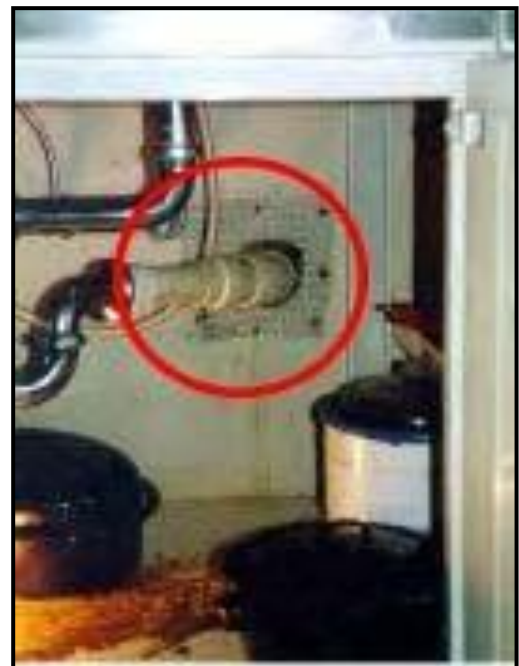
Use lath metal around pipes
